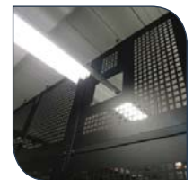
Access for existing lighting fixtures
