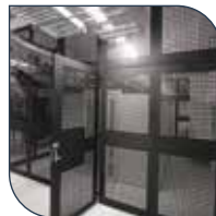
Large open mesh pattern to maximise airflow
