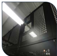
Access for existing lighting fixtures
