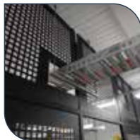
Cables into and out of data cage
