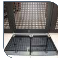
Data cage extends under flooring
