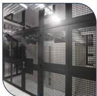
Large open mesh pattern to maximise airflow
