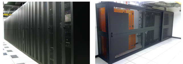
Top: Racks positioned and secured, ready for further on-site fit-out; Bottom Left: Completed cabinets; Bottom Right: Custom designed cage.
