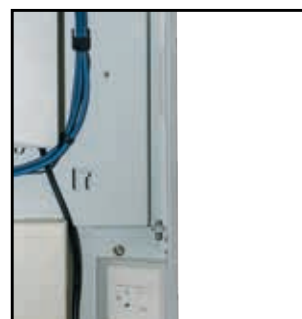
Hinged mounting pan allows easy access behind mounting pan to route fibre to NTD enclosure.
