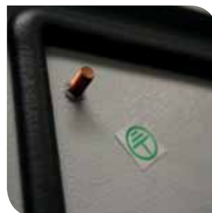
Earthing points for certification
