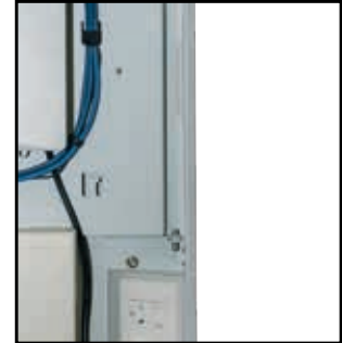
Hinged mounting pan allows easy access behind mounting pan to route fibre to NTD enclosure.
