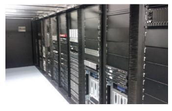
If you have already laid out your room in hot and cold aisles, with cabinets orientated 'front to front' and 'back to back', then you will achieve the best cooling by blocking unused panel spaces in your cabinets.
