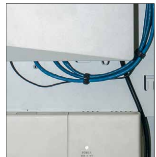
Power Supply Unit (not included) – Mounting position for NBN battery backup power supply.
