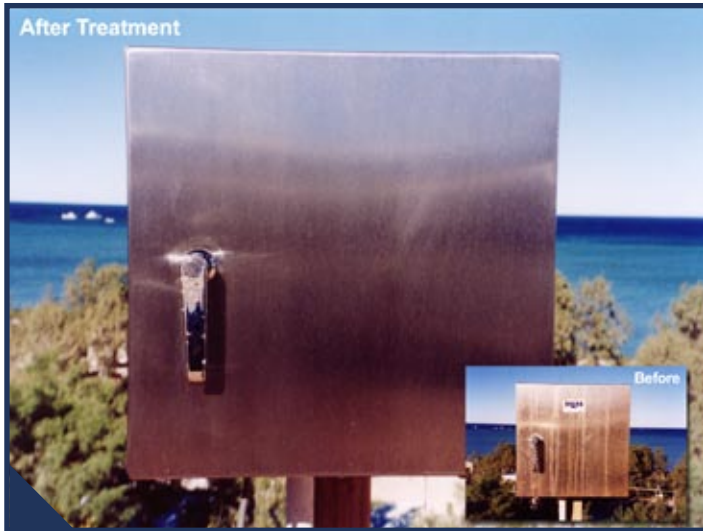
Figure 5 - Showing tea staining after treatment
